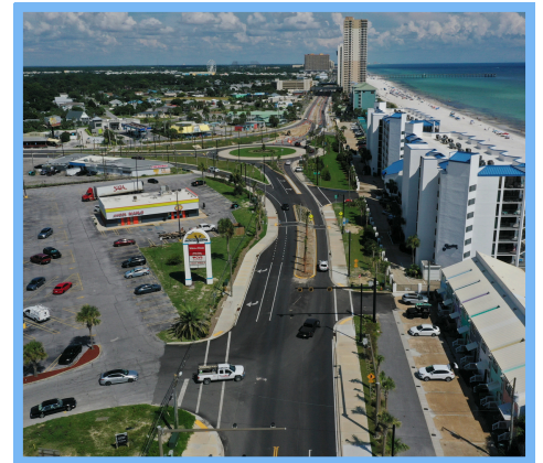
Looking east on Front Beach Road toward the roundabout.
